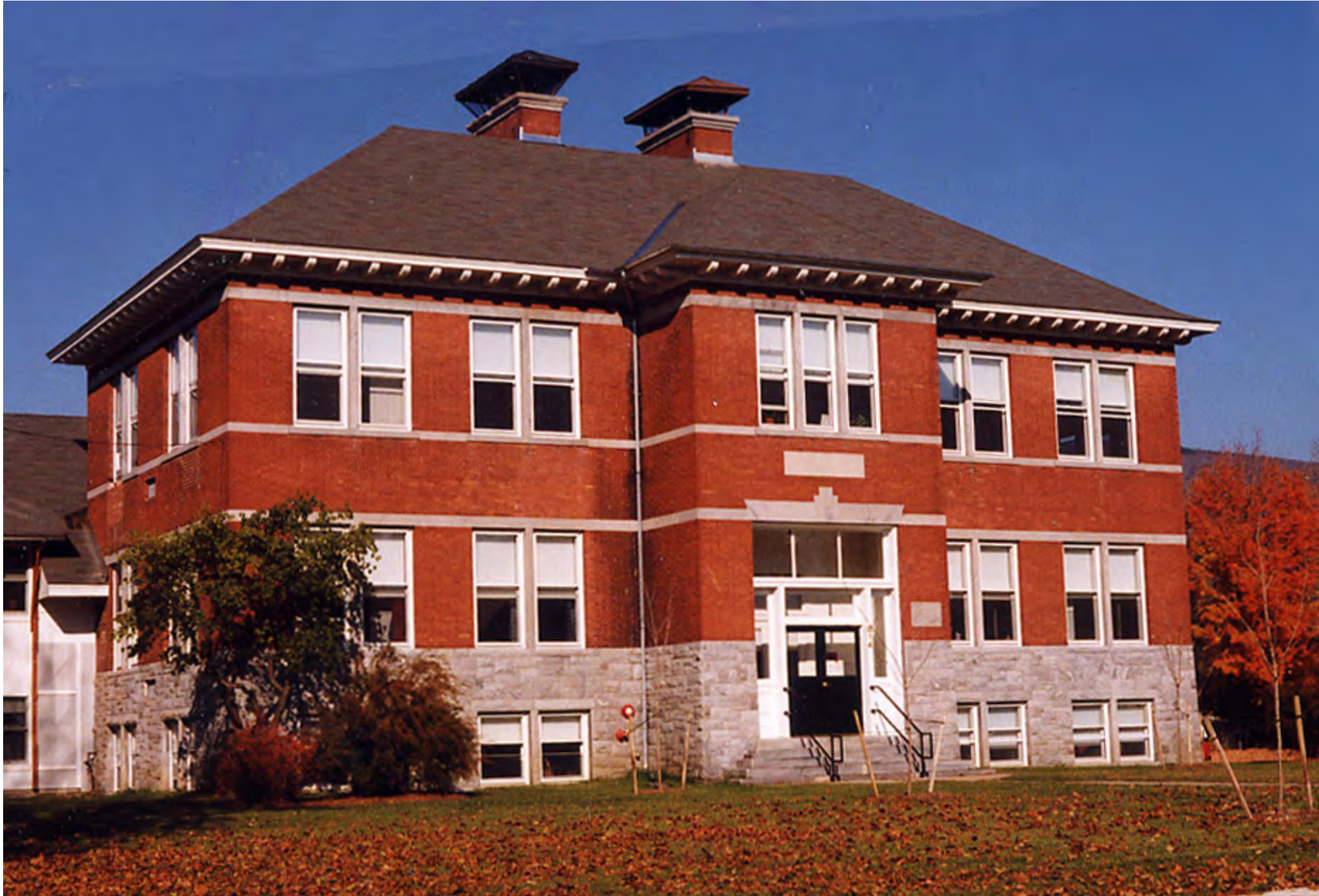
The Cora B. Whitney School in Bennington was redeveloped by Shires Housing to create 22 homes for seniors (13 affordable).
